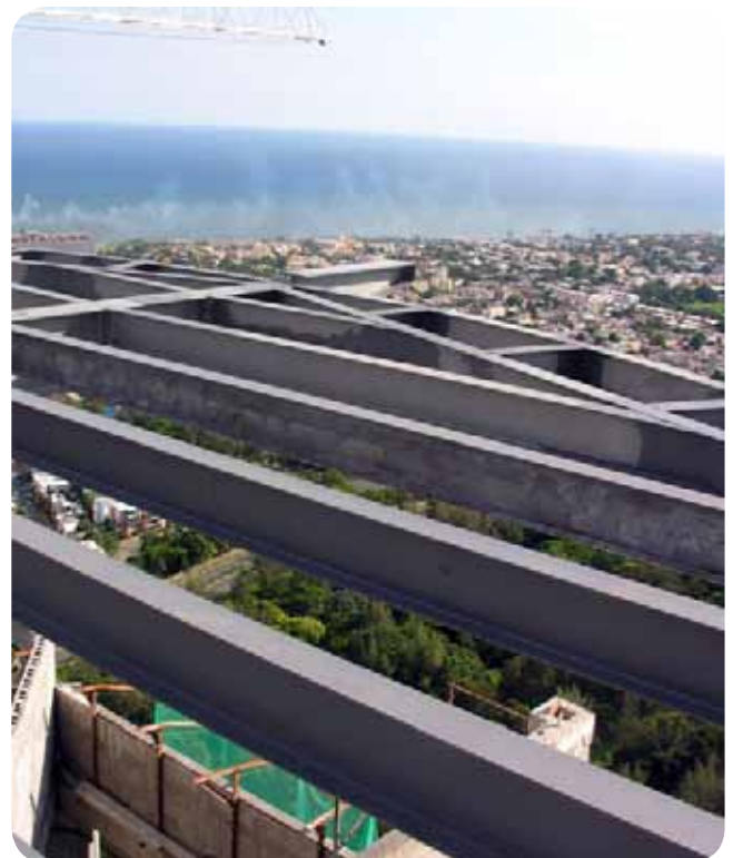
FRP is now being used in the construction of many different projects, like this helicopter landing platform
