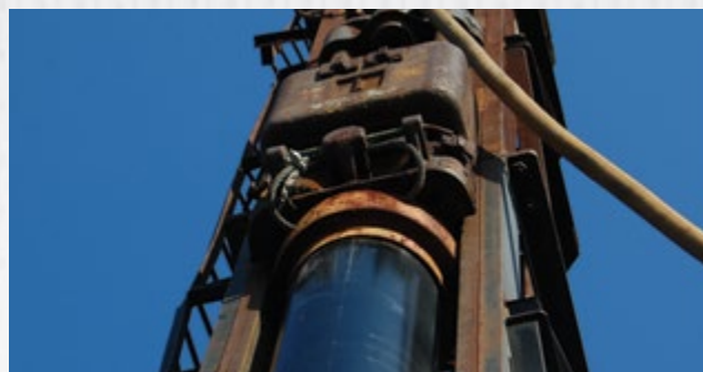
Vulcan 01 Impact Hammer Driving 16" Diameter SUPERPILE®
