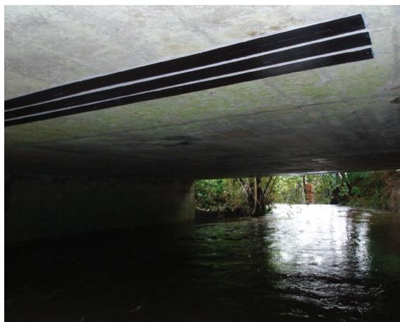
Figure 2.1 FRP edge beam strengthening (courtesy Atkins)
