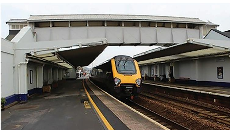
Grade II listed Victorian metallic footbridge, and was chosen for maximum durability in the very severe coastal environment. The bridge form comprised U-frame girders with GFRP roof and stairs. The Grading II listing meant that the new bridge had to look as similar as practical to the old metallic bridge, and aesthetic considerations necessitated the inclusion of features such as dome-headed bolts to look like rivets.
