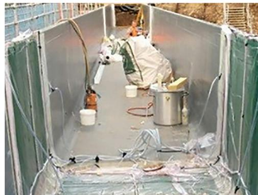
Figure 2.18 Site infusion (courtesy Delft Infra Composites)
