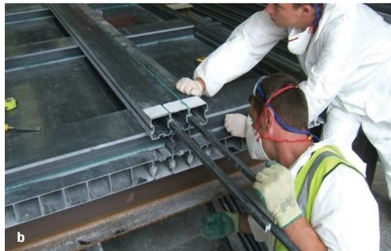
Figure 5.9 Mechanical interlock connection with pultruded ACCS as used in the St Austell footbridge, near St Austell, England (2007). Bridge cross-section (a), and assembling mechanical interlocking connection (b) (courtesy Brian Bell and Pipex PX)
