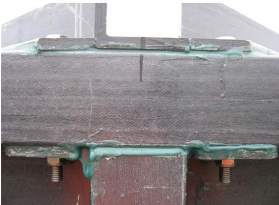
Figure 5.8 Hybrid bonded-bolted connection with pultruded shapes for the Launder Aqueduct, England (courtesy Brian Bell and Pipex PX)
