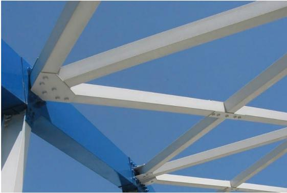
Figure 5.6 Typical bolted connections with pultruded shapes for the Lleida pedestrian bowstring bridge, Lleida, Spain (courtesy Fiberline Composites)
