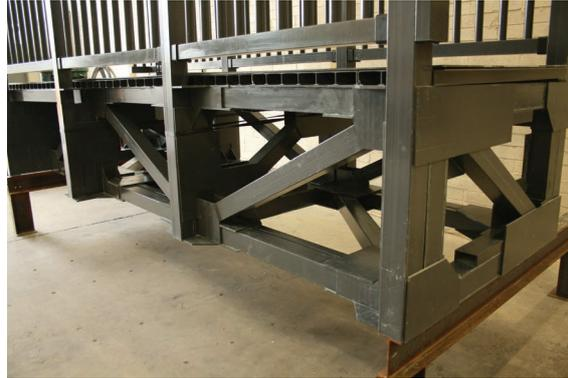
Figure 5.7 Bonded connections with pultruded shapes for the Leri footbridge, Borth, Wales (courtesy Brian Bell and Pipex PX)
